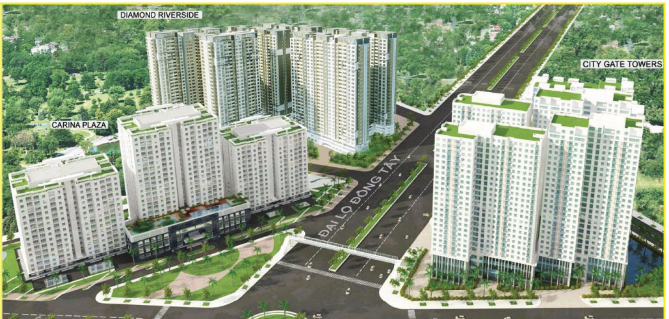
Dự án City Gate Tower - Tp.HCM
