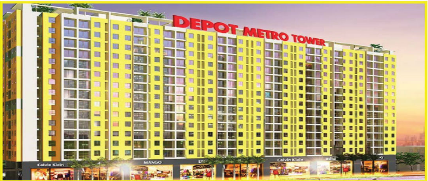
Dự án Depot Metro Tower
